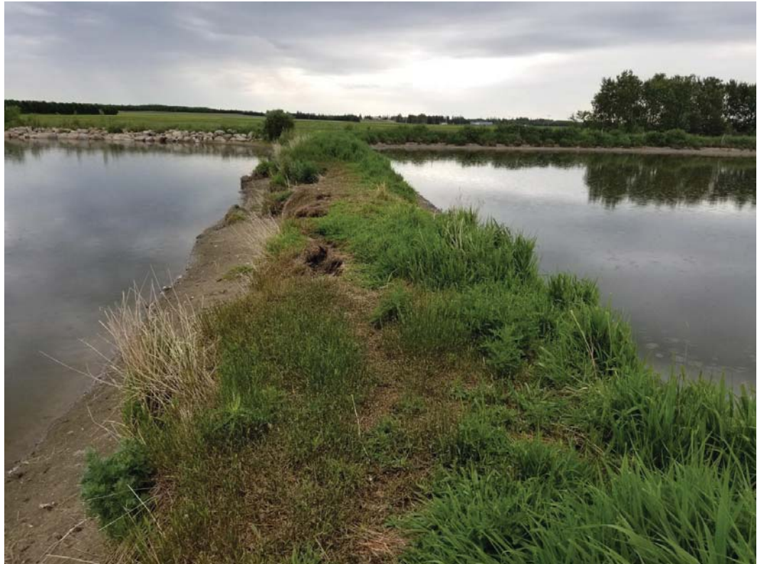
Figure 1 - Intercell dyke looking east
