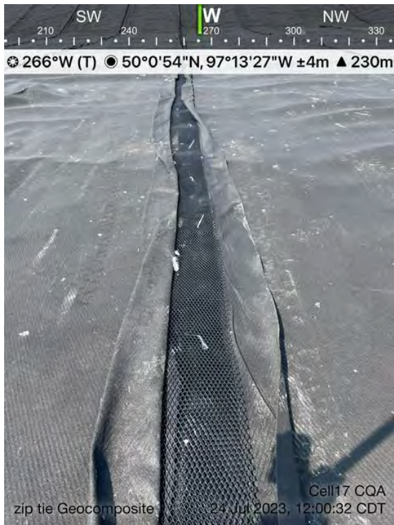
Geocomposite Seams Zip Tied
