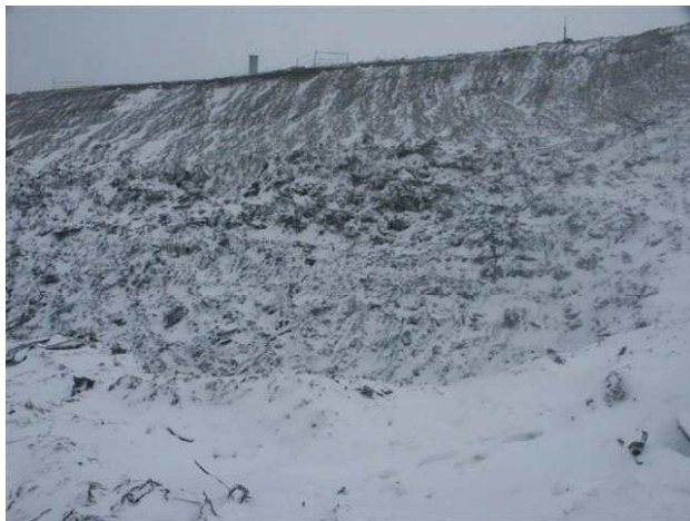
Figure 2. Slope steepened to 1H:1V
