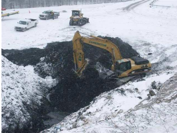
Figure 1. Excavation in progress at the south slope of Barrie landfill.
