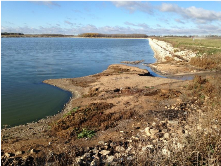
Photo 1. Truck unloading area at the west cell.
