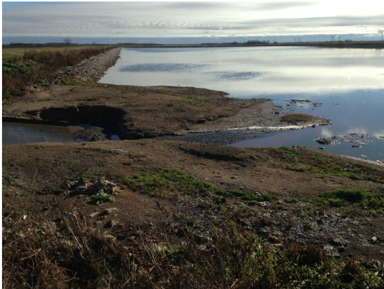
Photo 2. Truck unloading area at the east cell.
