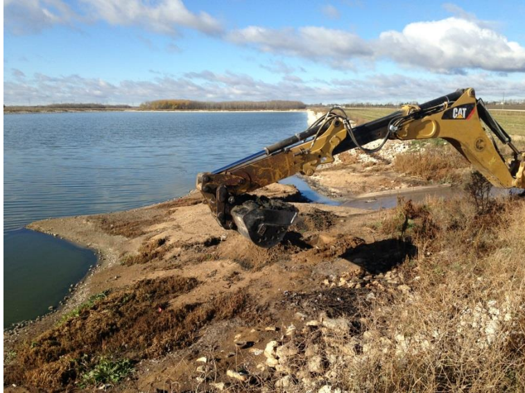
Photo 3. Sampling lagoon solids from west cell with back hoe.
