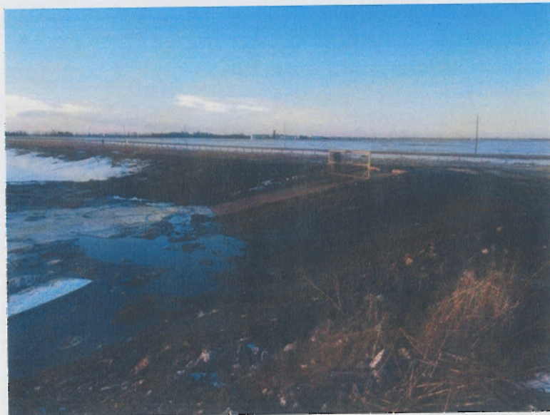
Photo 4. Completed west cell.
