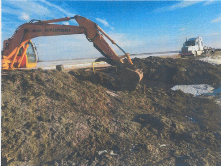
Photo 1. Excavation of dried solids for removal in east cell.
