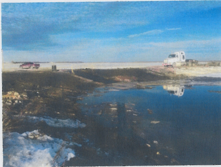
Photo 3. Completed east cell.
