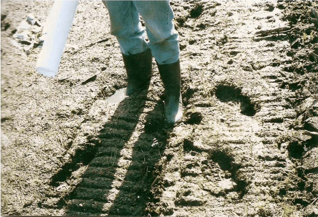
Plate 3: Saturated Condition of Winter Road
