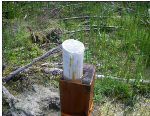
D. Flowing artesian conditions at MW-7-LS.
