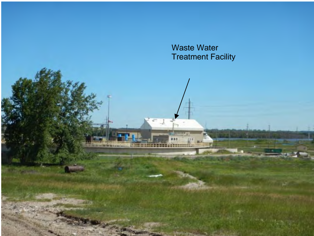
Photograph 8: Wastewater treatment facility located northeast of landfill (11-Jul-14).
