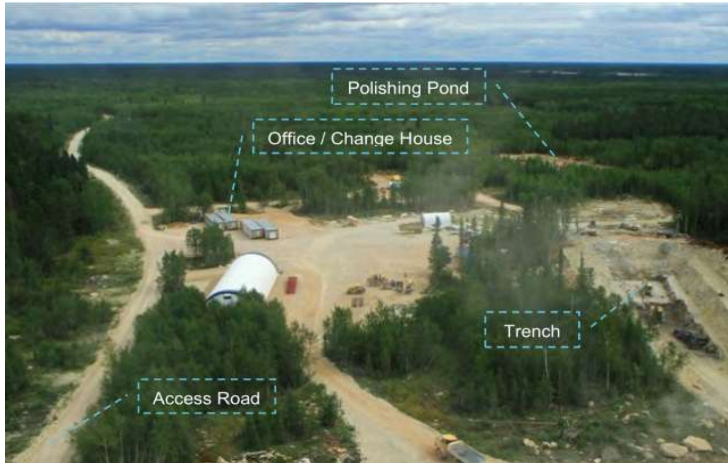
Reed AEP Site under Development, looking east (August 2012)
