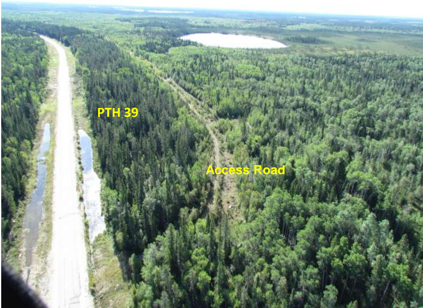
Looking East Toward AEP Site Along Existing Access Road (2011)
