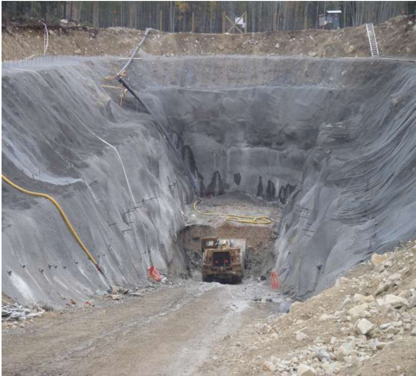
Trench Excavation – Fall 2012
