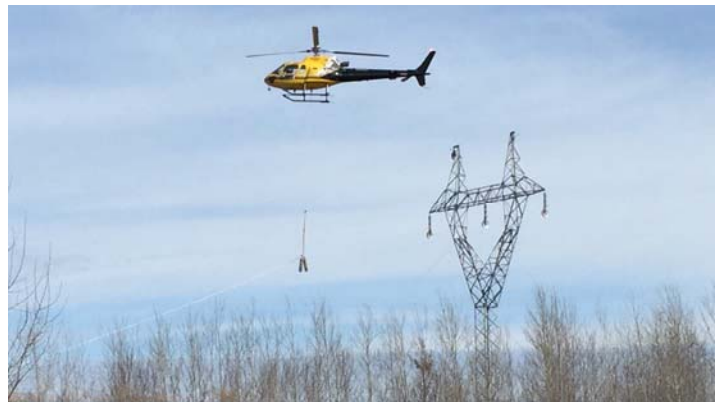
Photo 1: Construction crews used helicopters to install conductors in 2017/18
