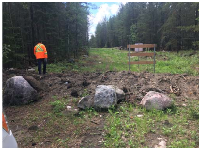
Photo 4: Access trail monitoring is continuing after decommissioning
