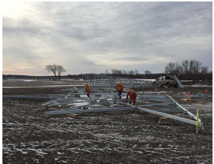
Photo 2: Final tower construction was completed in 2017/18
