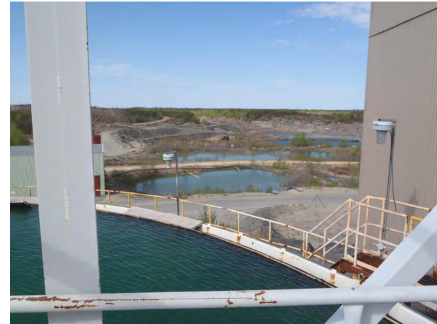
Chisel North WTP with Chisel Open Pit in Background
