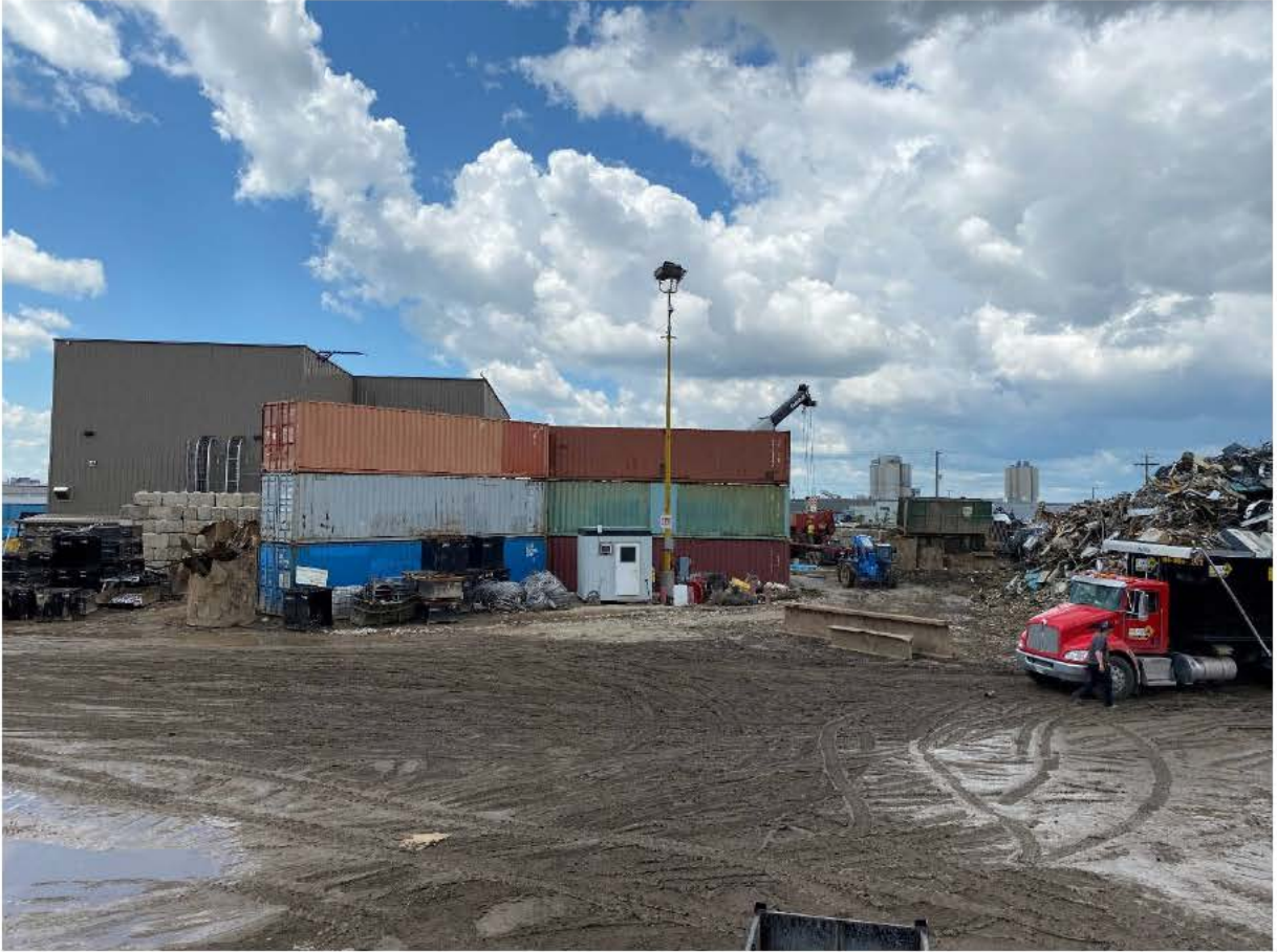
Figure 3: V-Shaped Noise Barrier Wall
