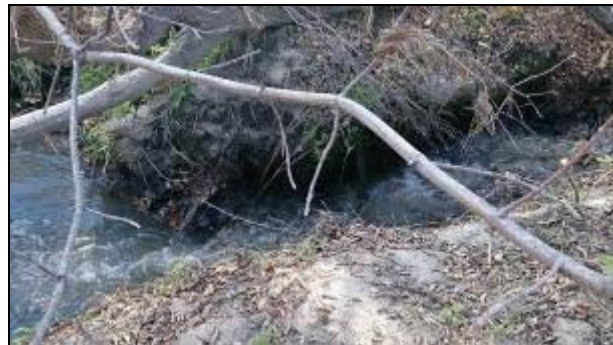
Photo 4-16: Discharge from effluent drainage channel into Gopher Creek.
