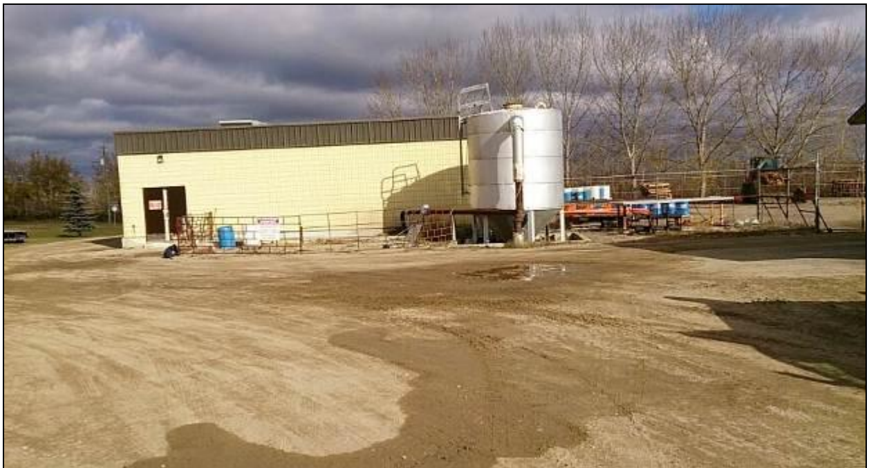
Photo 2-2: Southwest elevation of existing Virден WWTP.
