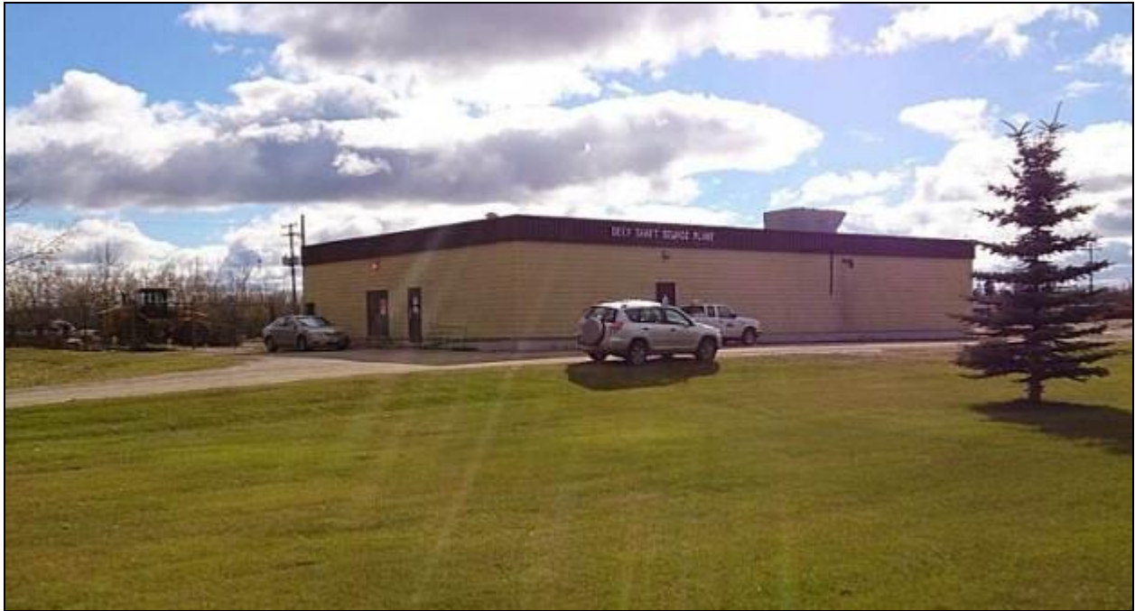
Photo 2-1: North elevation of existing Virден WWTP.
