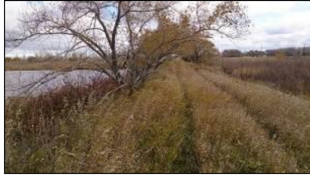
Photo 4-6: Dyke at south end of wetland.
