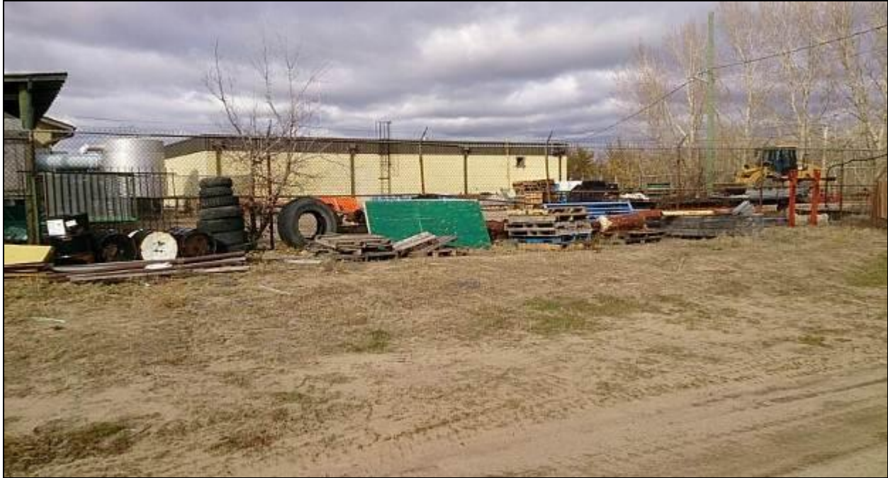
Photo 2-3: South elevation of existing Virден WWTP.
