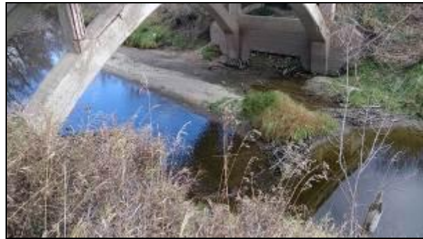
Photo 4-12: PR 257 bridge at Gopher Creek in Virден.
