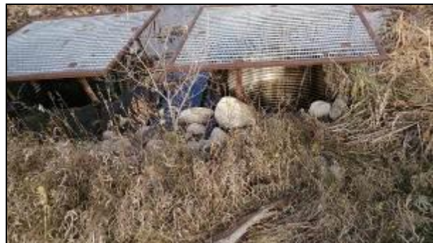
Photo 4-4: Inlet culverts on Bosshill Creek.
