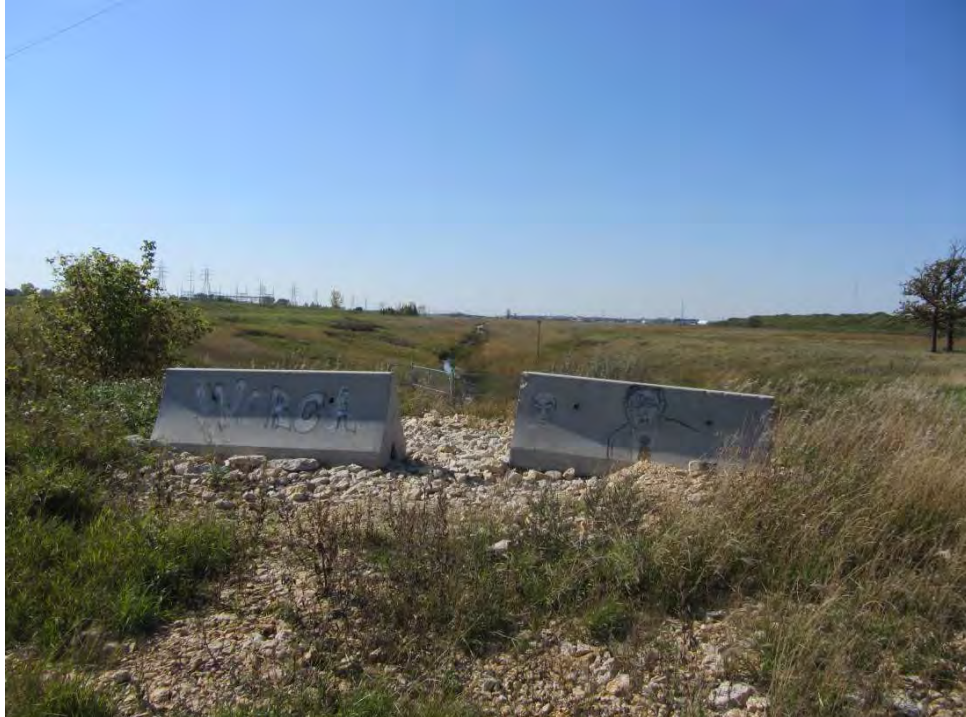
Photo 03. West view showing Lot 16 drain near Plaza Drive.
