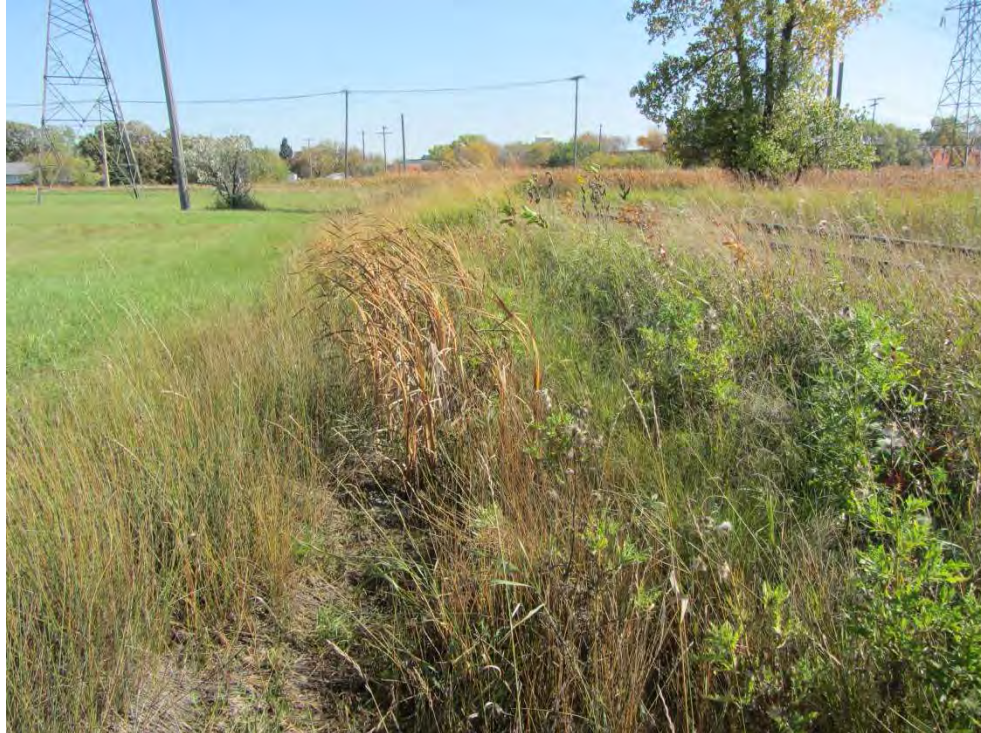
Photo 05. East view showing vegetation growing in ditch along side of railroad spur.
