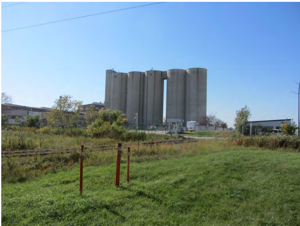
Photo 10. West view showing railroad spur and sugar storage silos.
