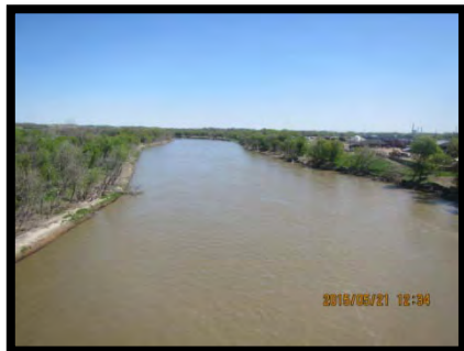
Photo 1 – Looking (east) downstream from Site#2582-00 on PTH 1A, May 21, 2015.
