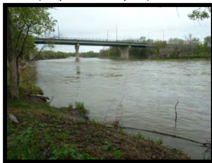
Photo 4 – Looking (west) at the east elevation, May 29, 2013 (Inspection Report).
