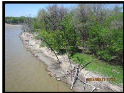
Photo 2 – Looking (northwest) at the northwest bank from structure, May 21, 2015.
