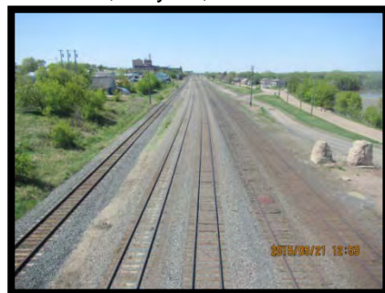
Photo 8 – Looking (west) at the CP rail, May 21, 2015.
