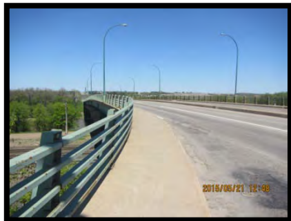
Photo 4 – Looking (north) at PTH 1A from the southwest abutment, May 21, 2015.
