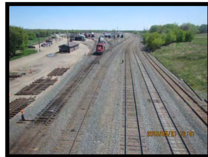
Photo 6 – Looking (east) at the CP rail (south of bank) from structure, May 21, 2015.
