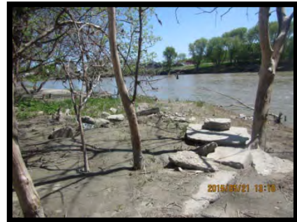
Photo 7 – Looking (east) at the northeast bank, May 21, 2015.
