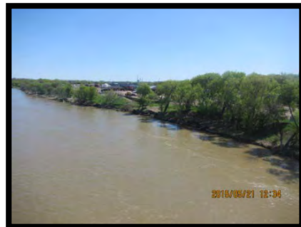
Photo 2 – Looking (southeast) at the southeast bank from structure, May 21, 2015.
