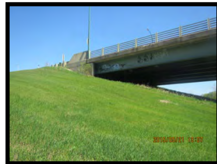
Photo 6 – Looking (northeast) at the northwest abutment, May 21, 2015.
