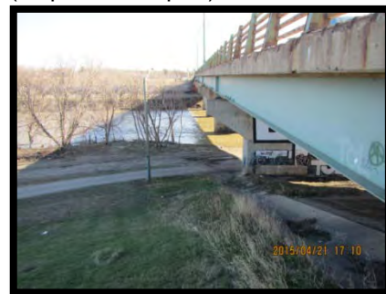
Photo 12 – Looking south from the northeast bank, April 21, 2015.
