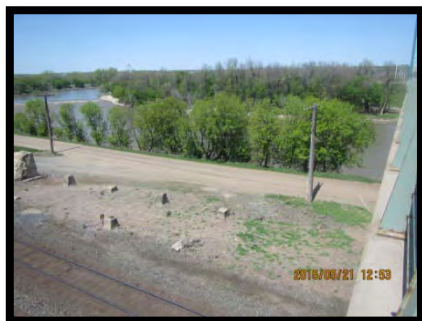
Photo 7 – Looking (northwest) at the CP road access and Assiniboine River bank, May 21, 2015.
