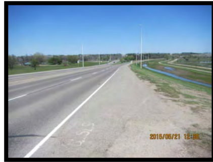
Photo 2 – Looking (north) at PTH 1A from structure, May 21, 2015.
