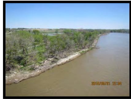
Photo 4 – Looking (northeast) at the northeast bank along the Assiniboine River from structure, May 21, 2015.
