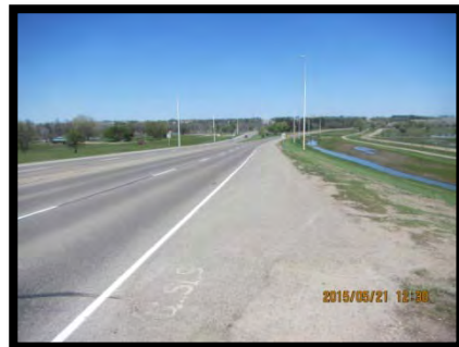
Photo 2 – Looking (north) at PTH 1A from structure, May 21, 2015.
