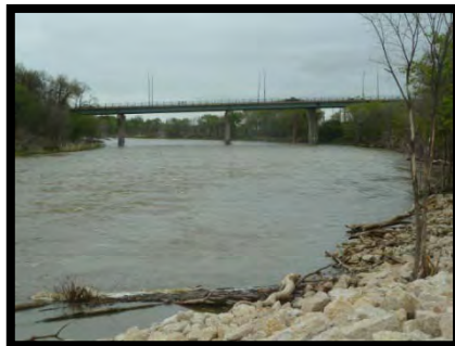
Photo 7 – Looking (east) at the west elevation, May 29, 2013 (Inspection Report).
