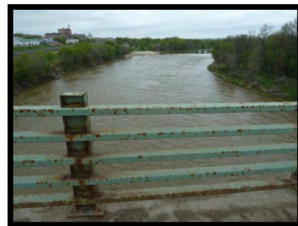
Photo 3 – Looking (west) upstream from structure, May 29, 2013 (Inspection Report).
