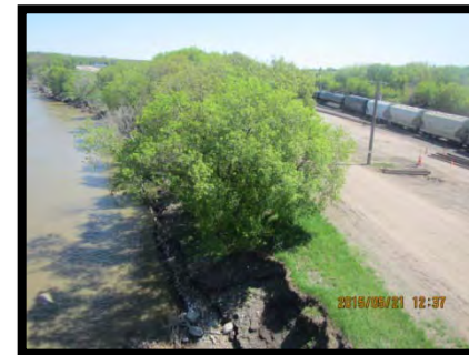
Photo 5 – Looking (east) along the southeast bank from structure, May 21, 2015.
