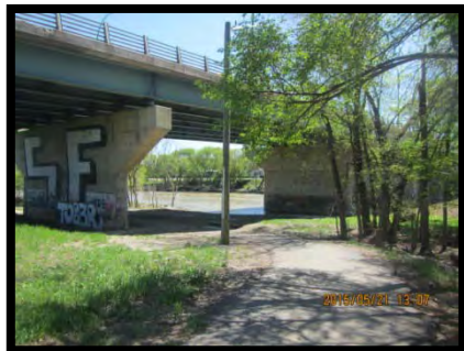
Photo 7 – Looking (south) at pedestrian path, structure and Assiniboine River, May 21, 2015.
