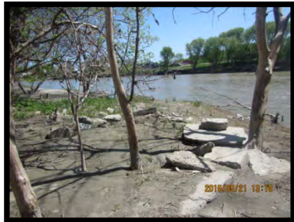
Photo 7 – Looking (east) at the northeast bank, May 21, 2015.
