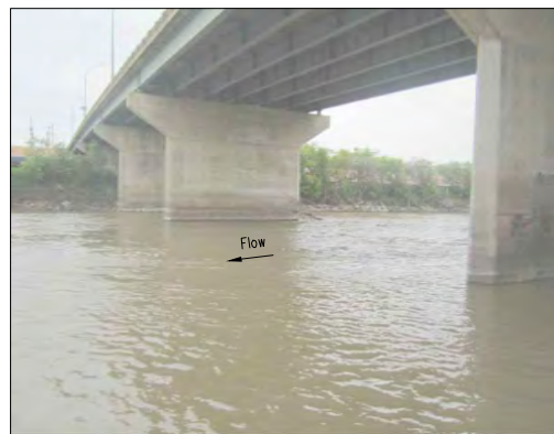
Photo 1 - Looking South (Upstream view of existing bridge) (2013)
