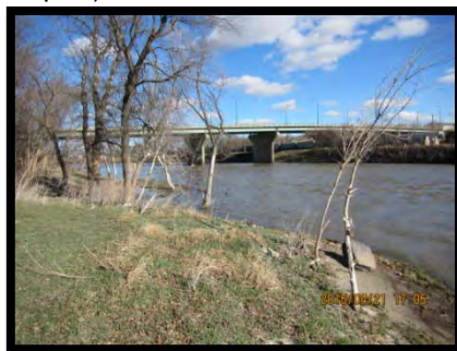
Photo 10 – Looking south east at Site#2582-00 from the northwest bank, April 21, 2015.
