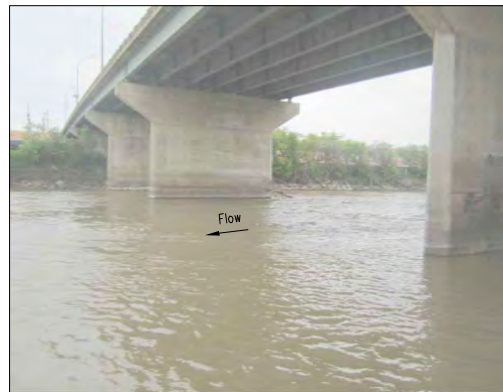
Photo 1 - Looking South (Upstream view of existing bridge) (2013)
