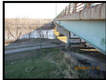
Photo 12 – Looking south from the northeast bank, April 21, 2015.
