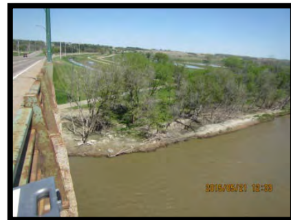
Photo 3 – Looking (northeast) at the northeast bank from structure, May 21, 2015.
