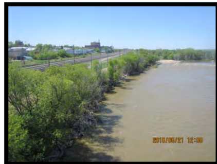
Photo 2 – Looking (west) at the southwest bank from structure, May 21, 2015.
