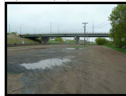
Photo 5 – Looking (west) at the east elevation, May 29, 2013 (Inspection Report).
