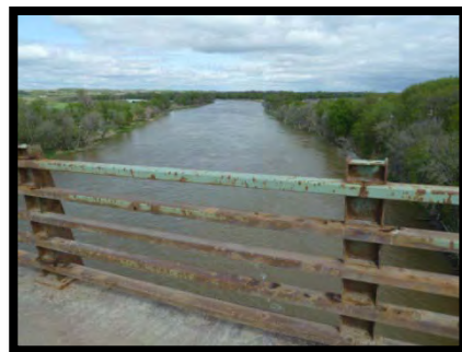
Photo 2 – Looking (east) downstream from structure, May 29, 2013 (Inspection Report).
