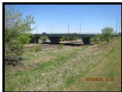
Photo 11 – Looking (northeast) at the upstream elevation (approx. 50 m west), May 21, 2015.
