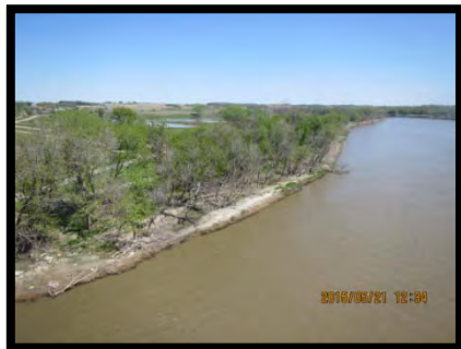
Photo 4 – Looking (northeast) at the northeast bank along the Assiniboine River from structure, May 21, 2015.
