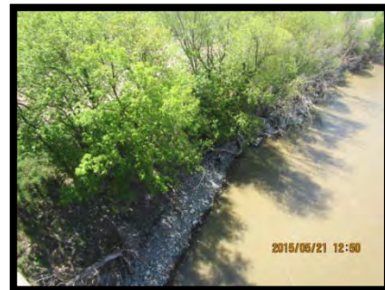
Photo 3 – Looking (southwest) at the southwest bank from structure, May 21, 2015.
