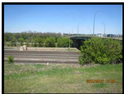
Photo 10 – Looking north at the upstream elevation, May 21, 2015.
