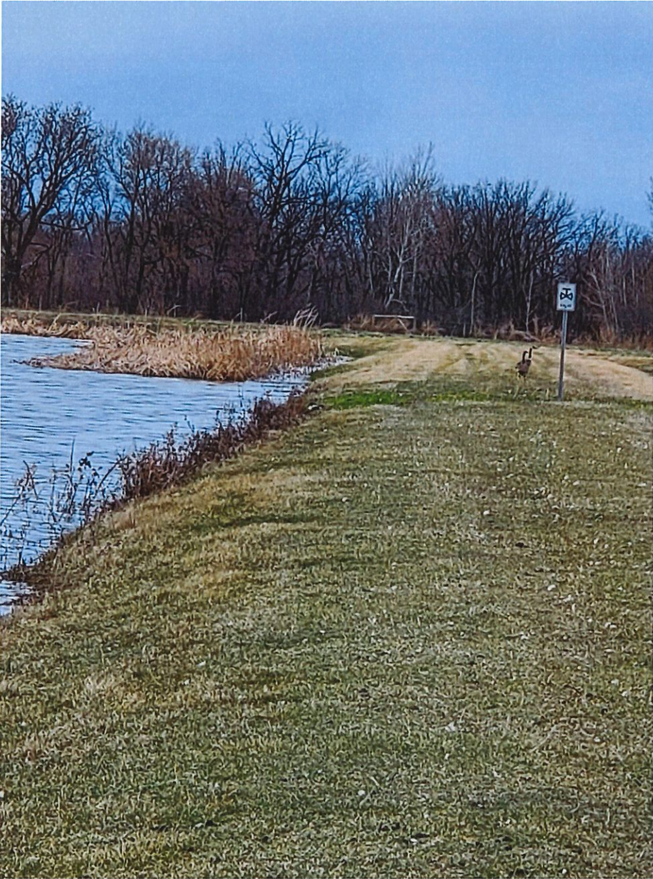
Photo 2. Second cell (old secondary cell)
