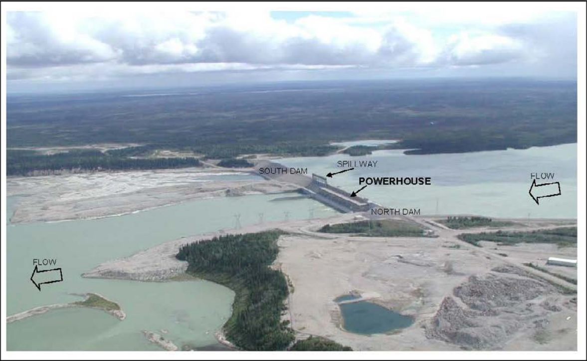
Figure 2: Photograph of Limestone Generating Station
