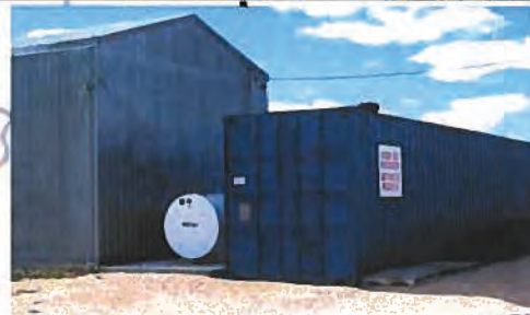
Tank on a pad and sea container – sampling Stonewall
