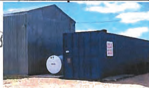
Tank on a pad and sea container – sampling Stormwater
