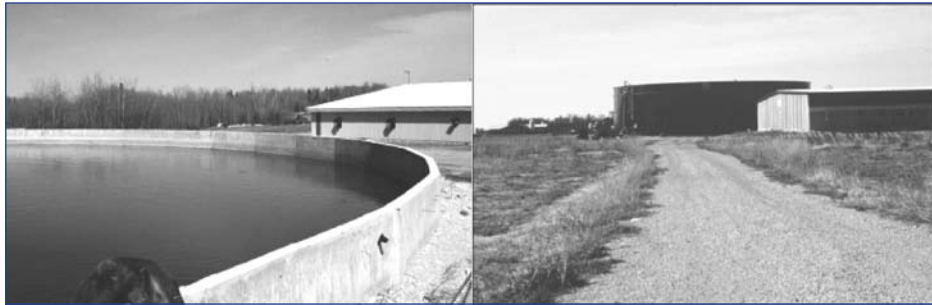
Concrete (left) or steel (right) liquid manure storage structures
