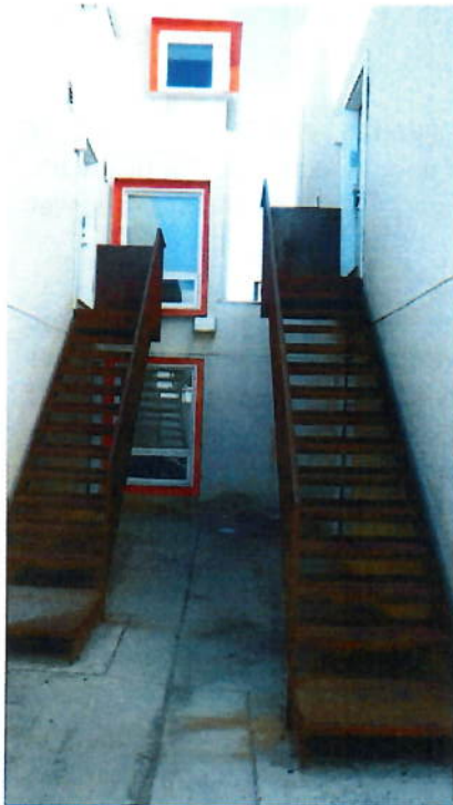
Fig. 18: A typical secluded entrance way where a security assessment may prove beneficial.
