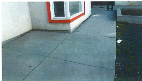
Fig. 1.: Jacking corner of Bldg A (unit a8).
