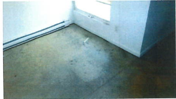
Fig. 16: Interior view of cantilever.
